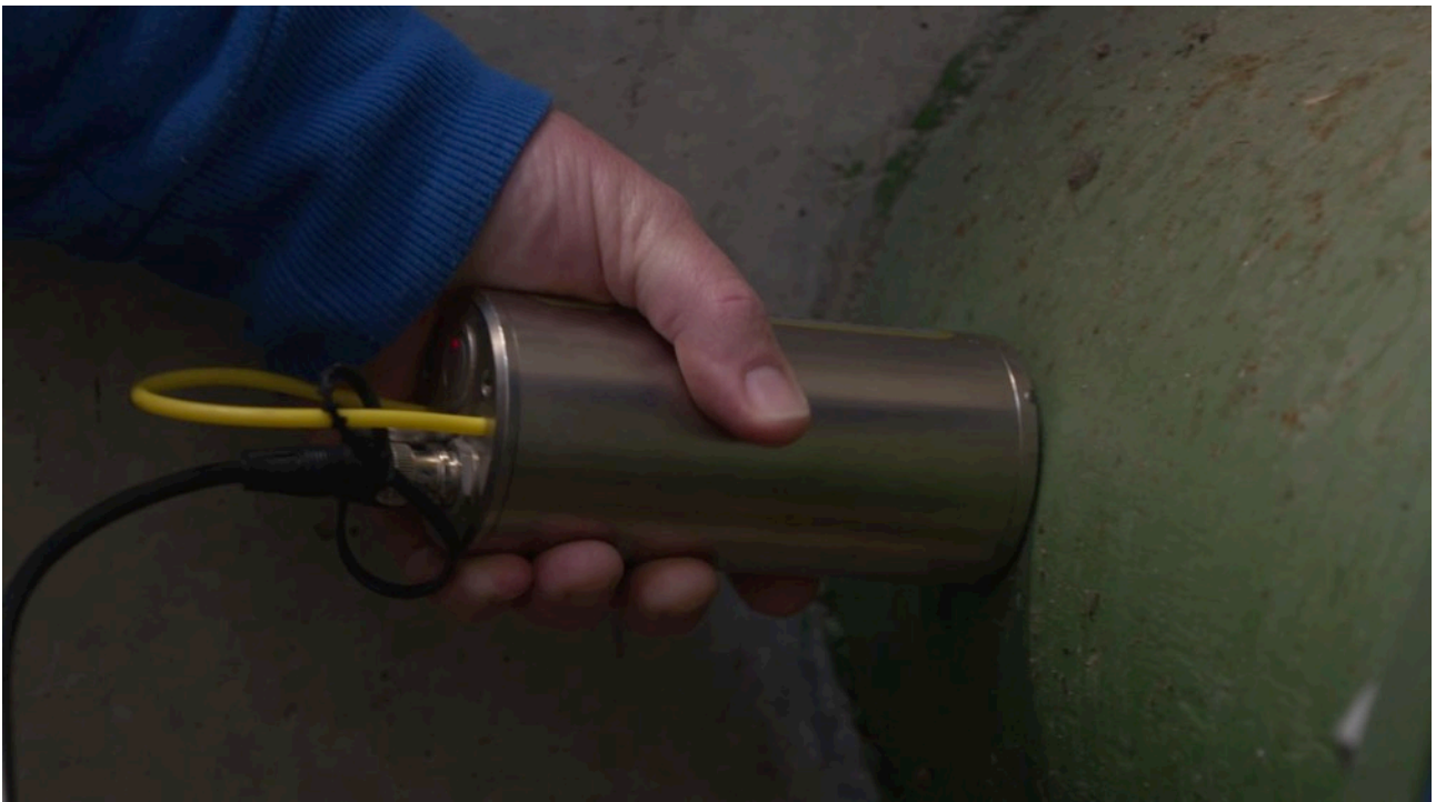
Figure 2.1 Frame of WADI VNR showing the acoustic method for water leak detection
