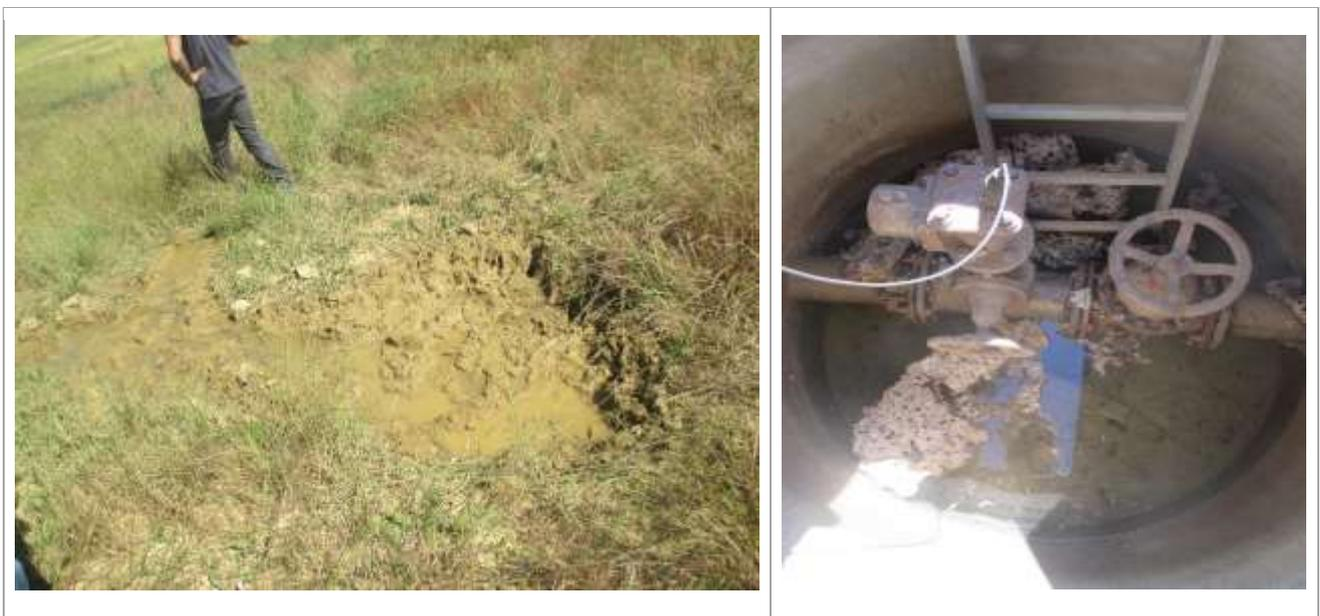
Figure 49 : Puddle between the drain valve and the connecting manhole, and drowned manhole
