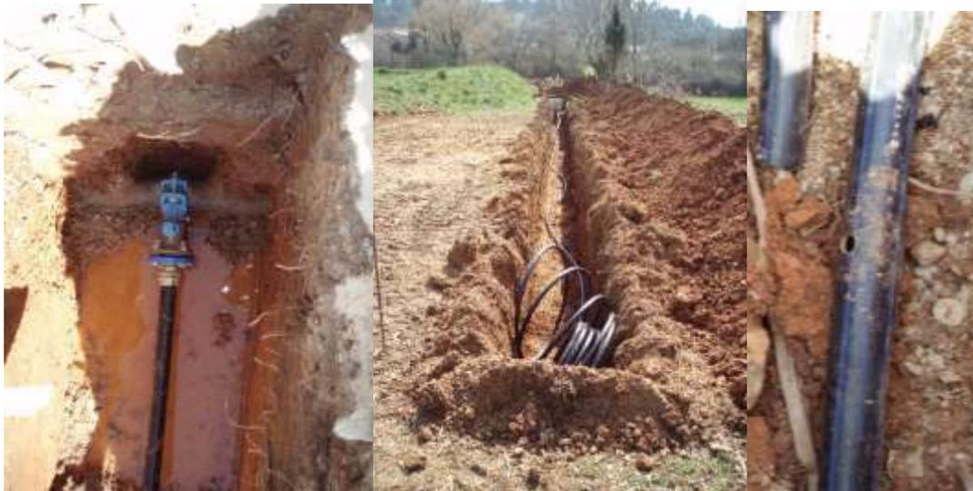
Figure 14: Artificial water leaks works : connection with existing pipe, trench for new pipe, hole for leak.
