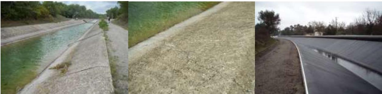
Figure 6: St Maximin open channel before and after refurbishment.
