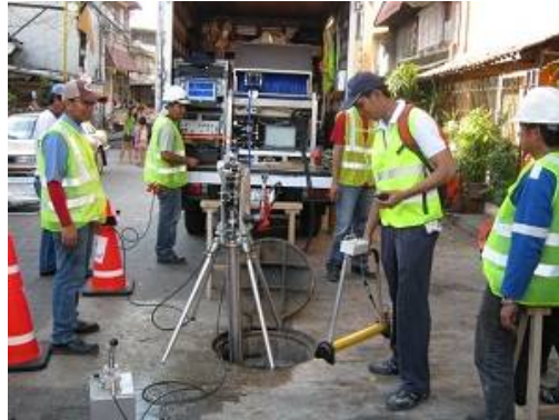
Figure 1-13 Engineers deploying the Sahara® tool inside a water main 7
