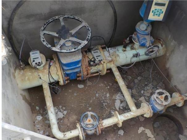
Figure 6.4 Pressure loggers at the boundary valve between sectors 3 and 4
