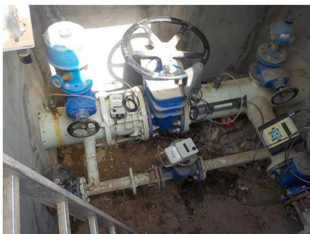
Figure 6.3 Pressure loggers at the boundary valve between sectors 1 and 2.
