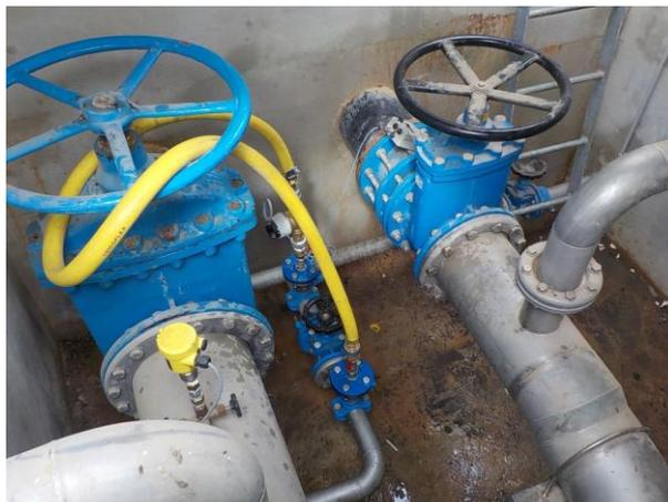
Figure 6.2 Installation of water meter to measure outflow from Clau des Lamberts SR.
