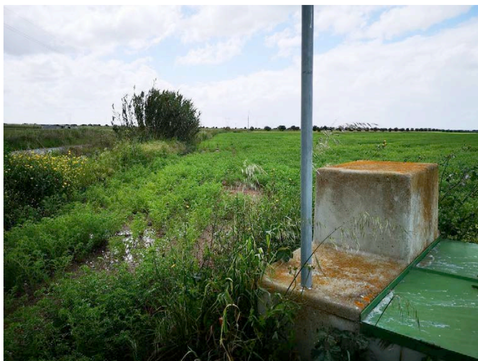
Figure 109 : Ferreira area. Photo of hydrant H9.6 taken on April 16, 2020 in west direction (H9.7 is at background on the top of the picture).
