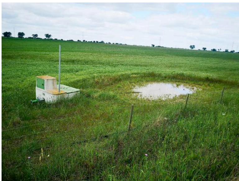
Figure 100 : Ferreira area. Photo of Hydrant H12.20 taken on April 16, 2020 in north direction.
