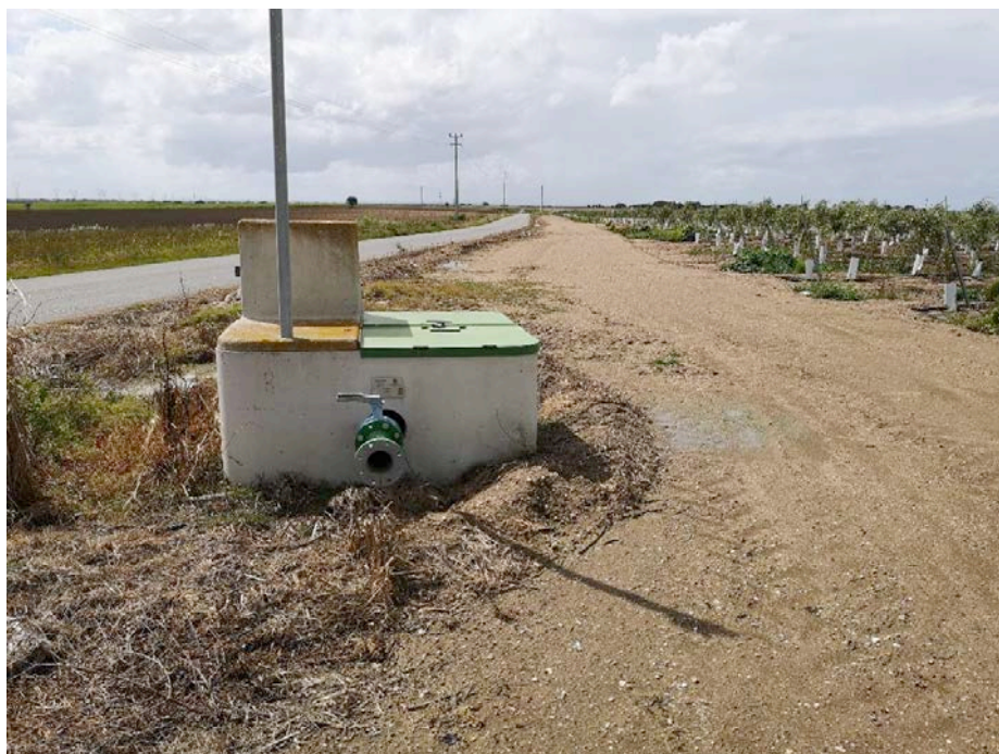
Figure 111 : Ferreira area. Photo of hydrant H9.10 taken on April 16, 2020 in west direction.
