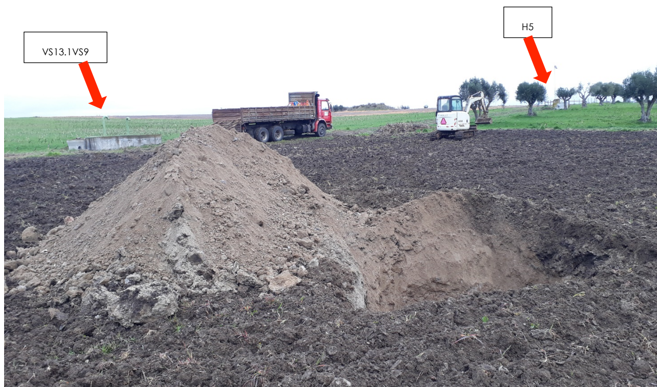
Figure 81 : Picture of the area close to the air valve VS13.1VS9, which is located in the concrete block at left. After the WADI airborne campaign, EDIA dug the soil a few tens of meters south of VS13.1VS9, in the zone corresponding to “real 1”. Below the surface, the soil was found dry as seen on the picture. Hence, the high water index in the zone “real 1” in Figure 69 and Figure 80 cannot be attributed to a real leak originating from the pipe at air valve VS13.1VS9.
