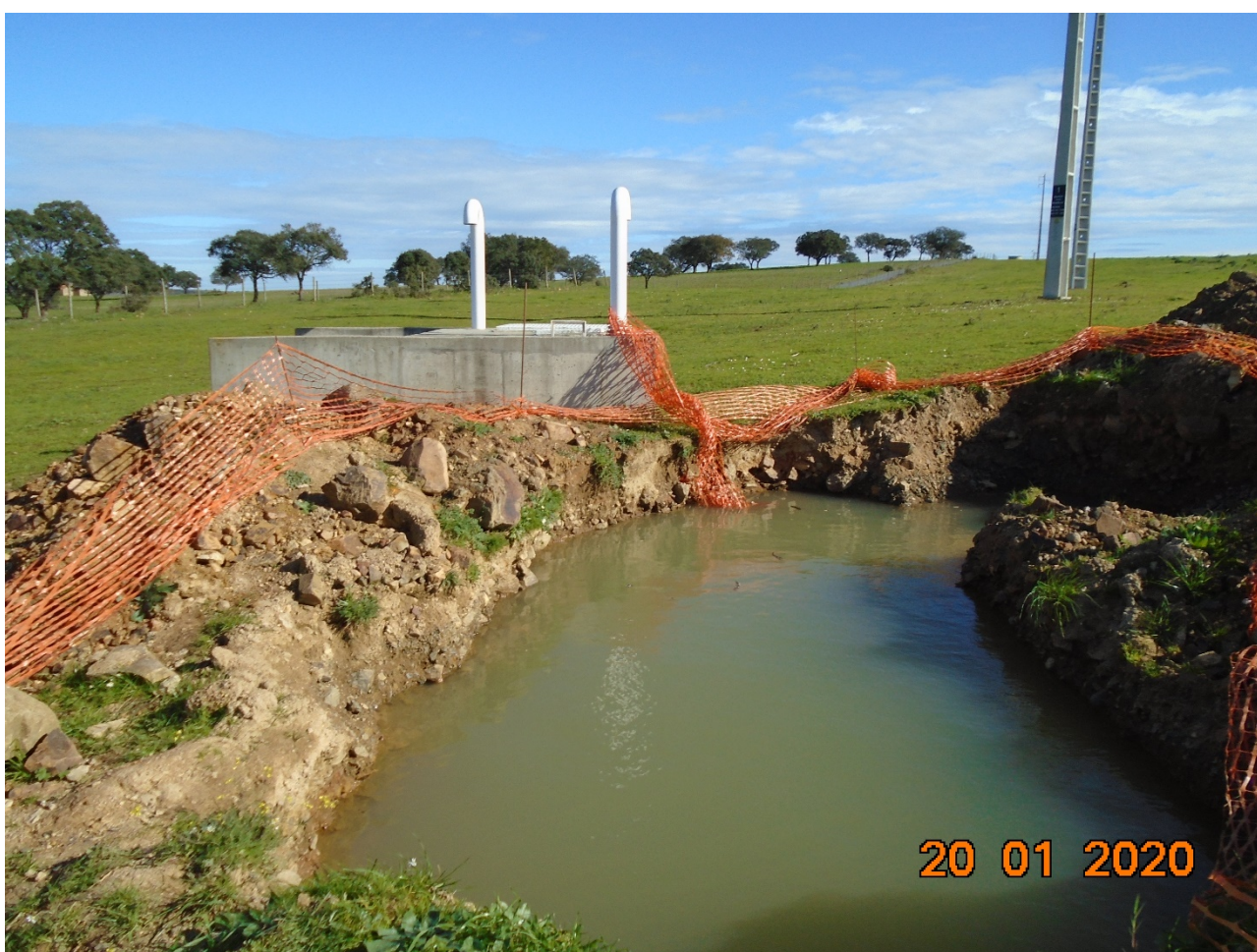
Figure 87 : Picture of the area close to the air valve north east of the reservoir.
