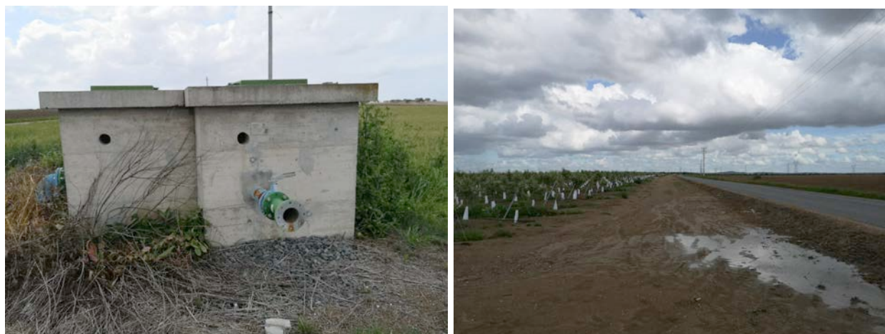
Figure 113 : Ferreira area. Photos of hydrant H9.11 taken on April 16, 2020 in west and east directions. The hydrant was not used for irrigation during last campaign. The right picture shows the drip lines of the olive plantation which always lead to water accumulation in the lower spots.
