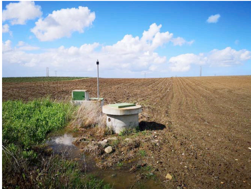
Figure 117 : Ferreira area. Photo of hydrant H17.4 taken on April 16, 2020 in north direction.
