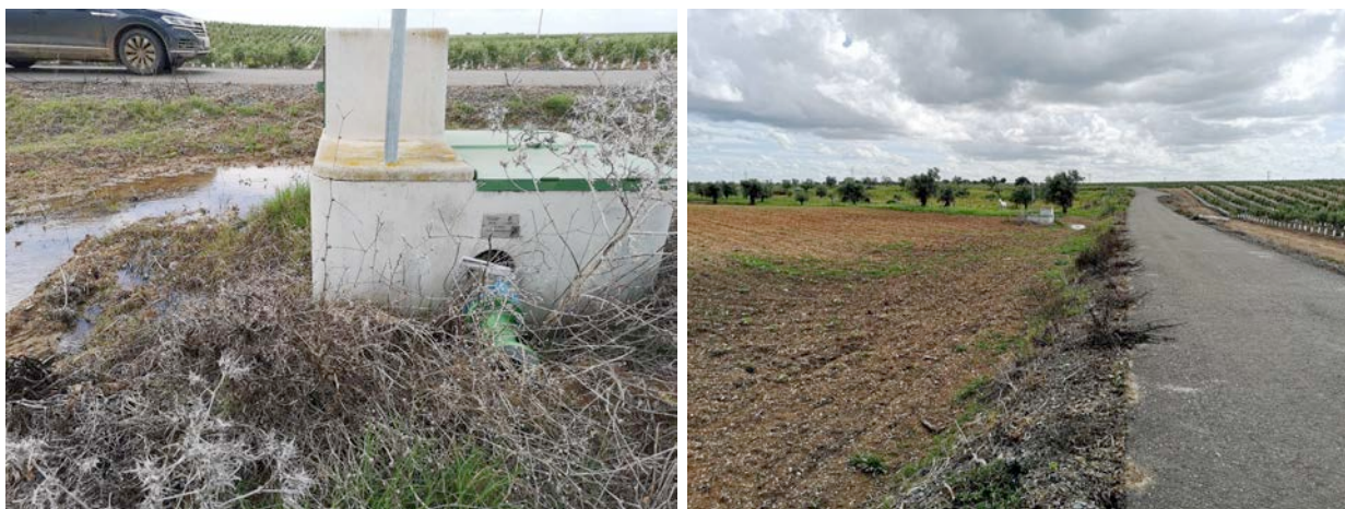
Figure 115 : Ferreira area. Photos of hydrant H9.18 taken on April 16, 2020 in northwest and southwest directions.
