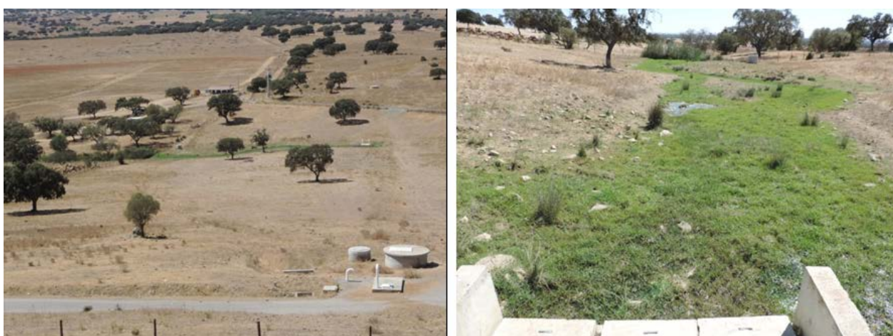
Figure 53: Vale de Gaio “natural leak” 2, west from the reservoir. Leak as seen from the reservoir (left) and close up of the leak (right).
