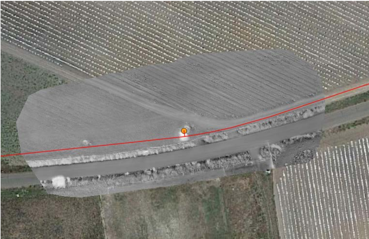
Figure 138 : Ferreira area. Artificial "leak" H9.7, Sept 12.
